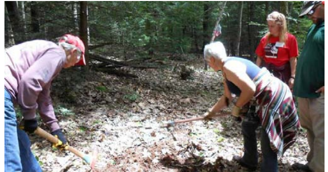
Work at the Pennsylvania Trails Seminar. Removing "duff" from the trails. This organic material (decayed leaves, etc.) absorbs and holds water on the trail.
